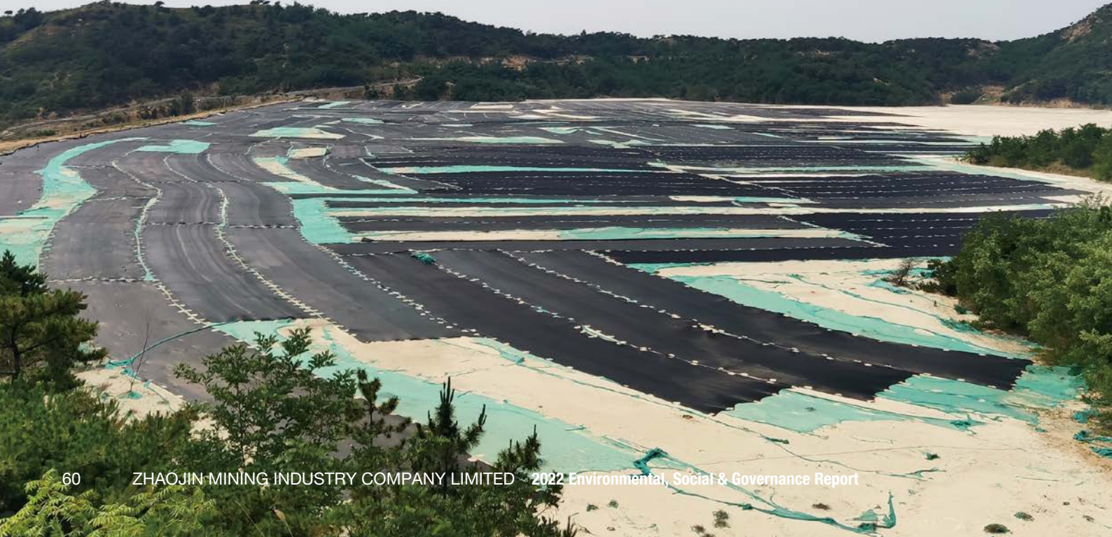
The picture shows the dust control netting in the storage area of the tailing pond, which can effectively reduce dust pollution
