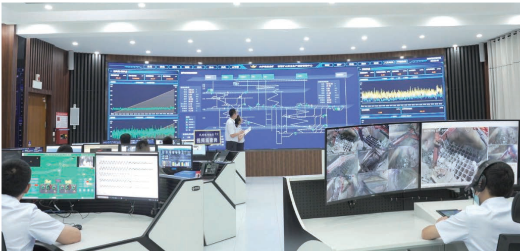
Production Dispatching and Command Center of Dayingezhuang Gold Mine
